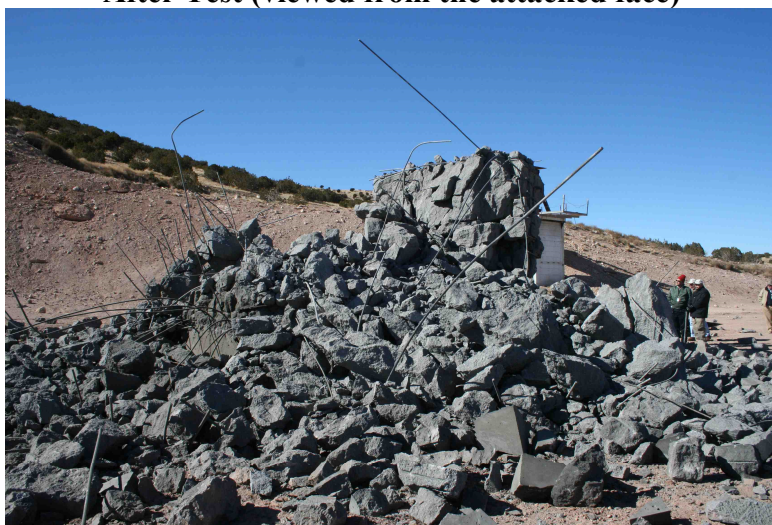
After Test (viewed from the attacked face)
