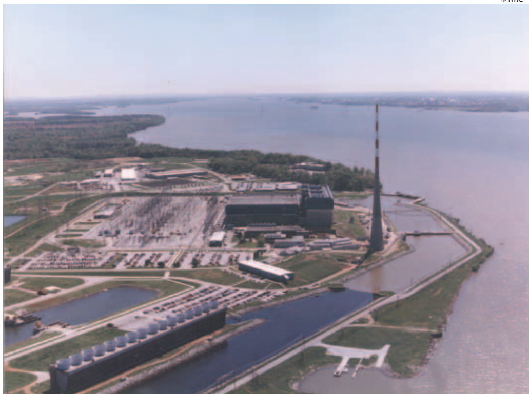
A serious fire at Alabama's Browns Ferry nuclear plant spurred the NRC to issue fire protection regulations in 1980 (and again in 2004), but more than three dozen reactors still do not comply.
